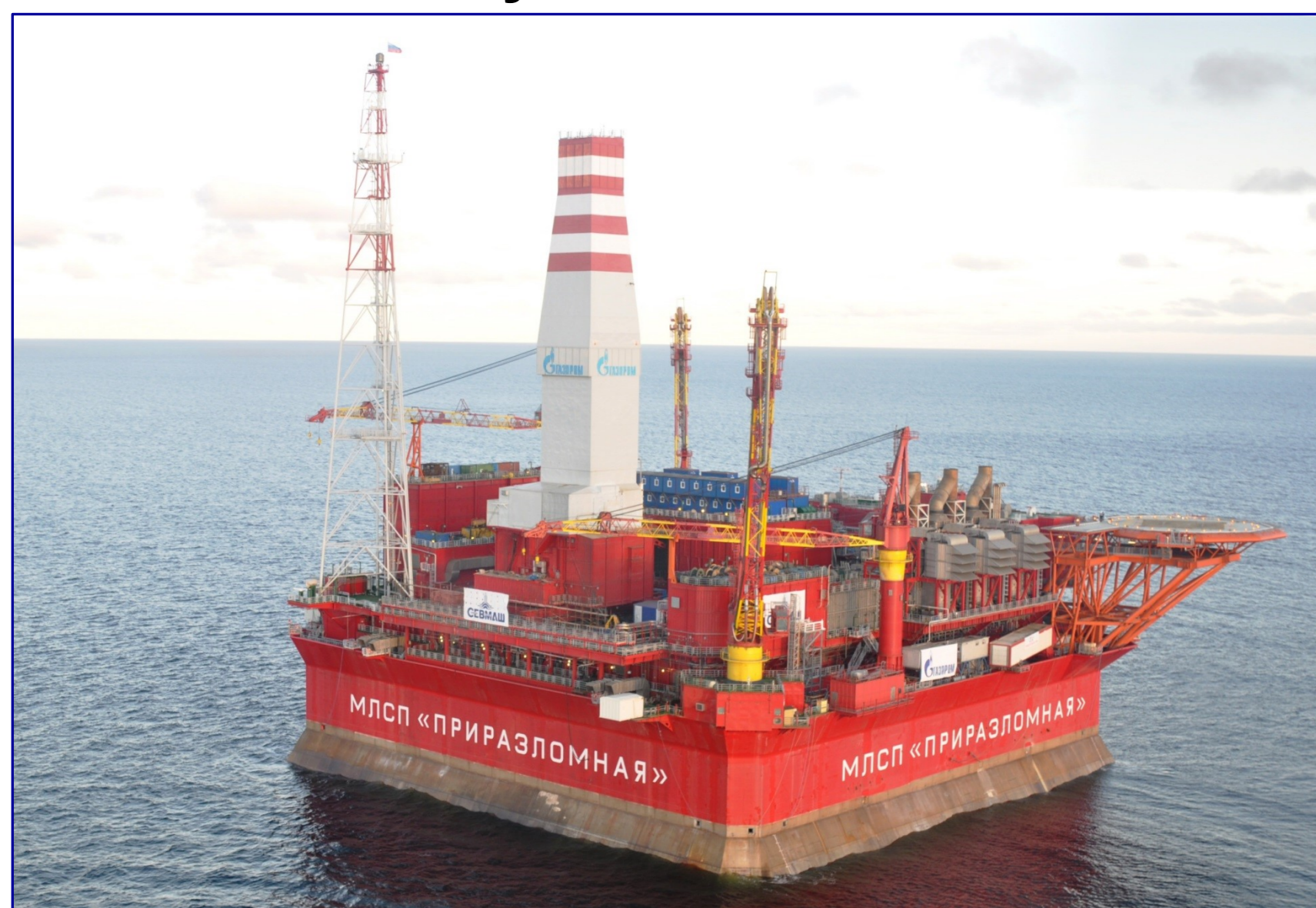
The Prirazlomnaya offshore ice-resistant oil-producing stationary platform
